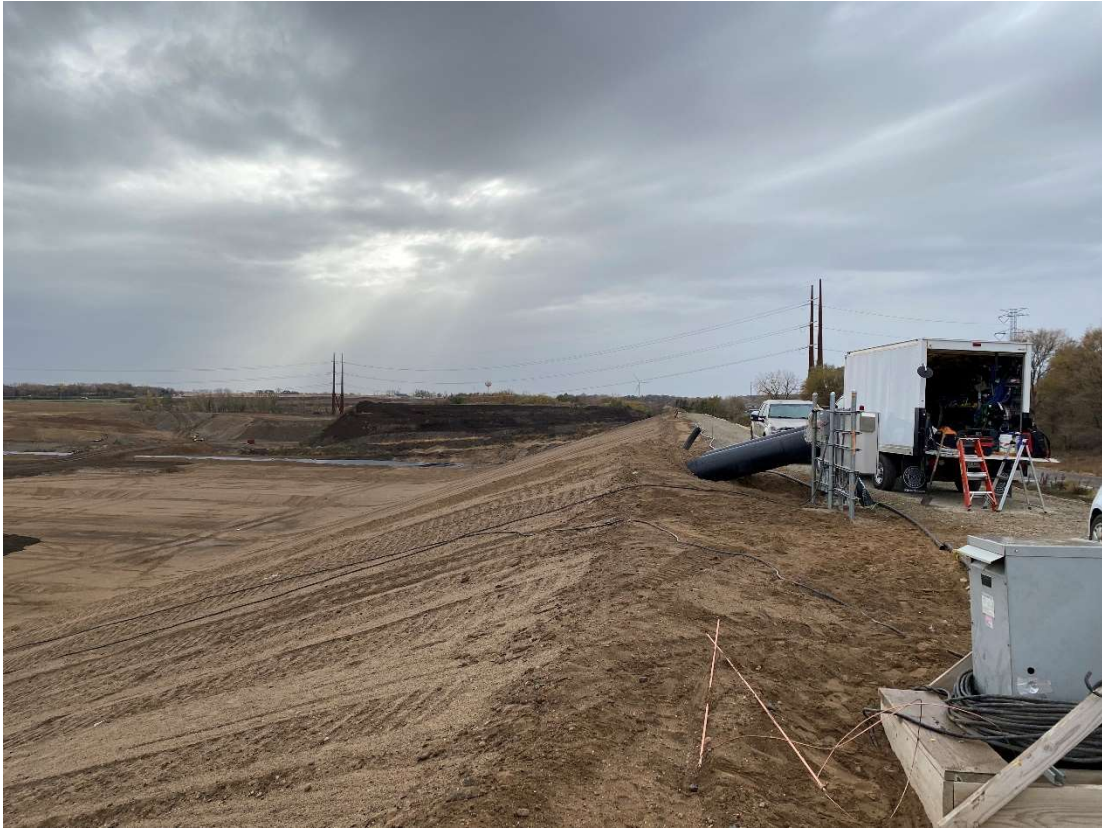
Location 13 – Cell 6A northwestern top of berm, looking southwest
