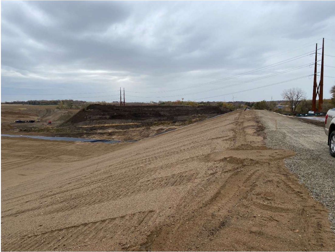
Location 12 – Cell 6A midpoint of northwestern inner berm, looking southwest
