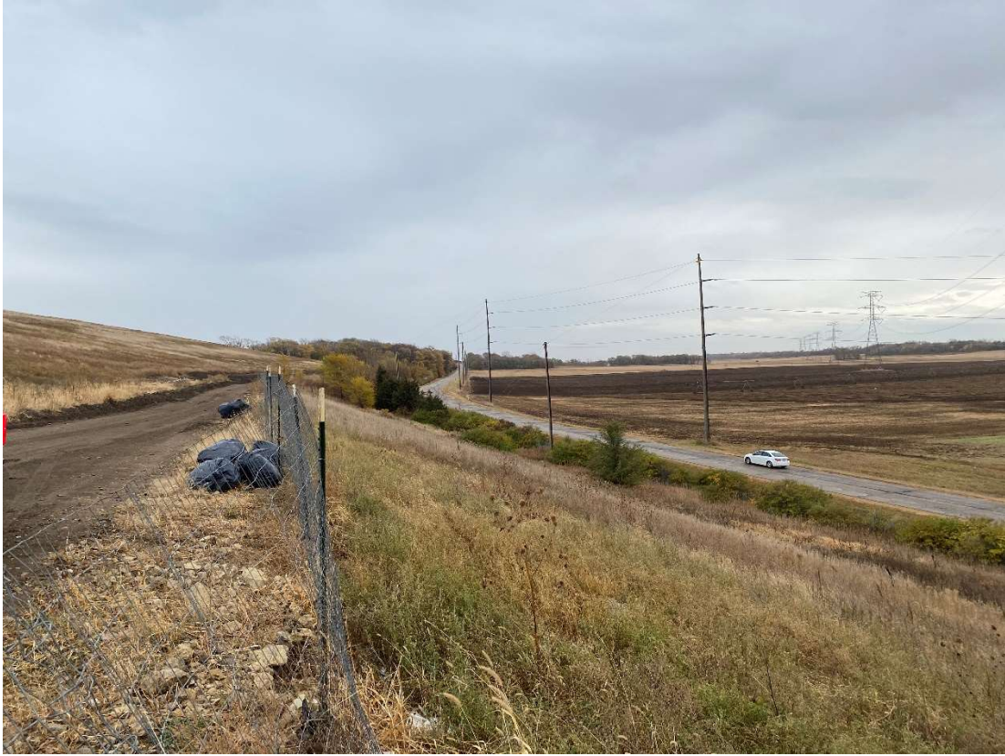
Location 7 – Cell 6D, midpoint of outer berm, looking east
