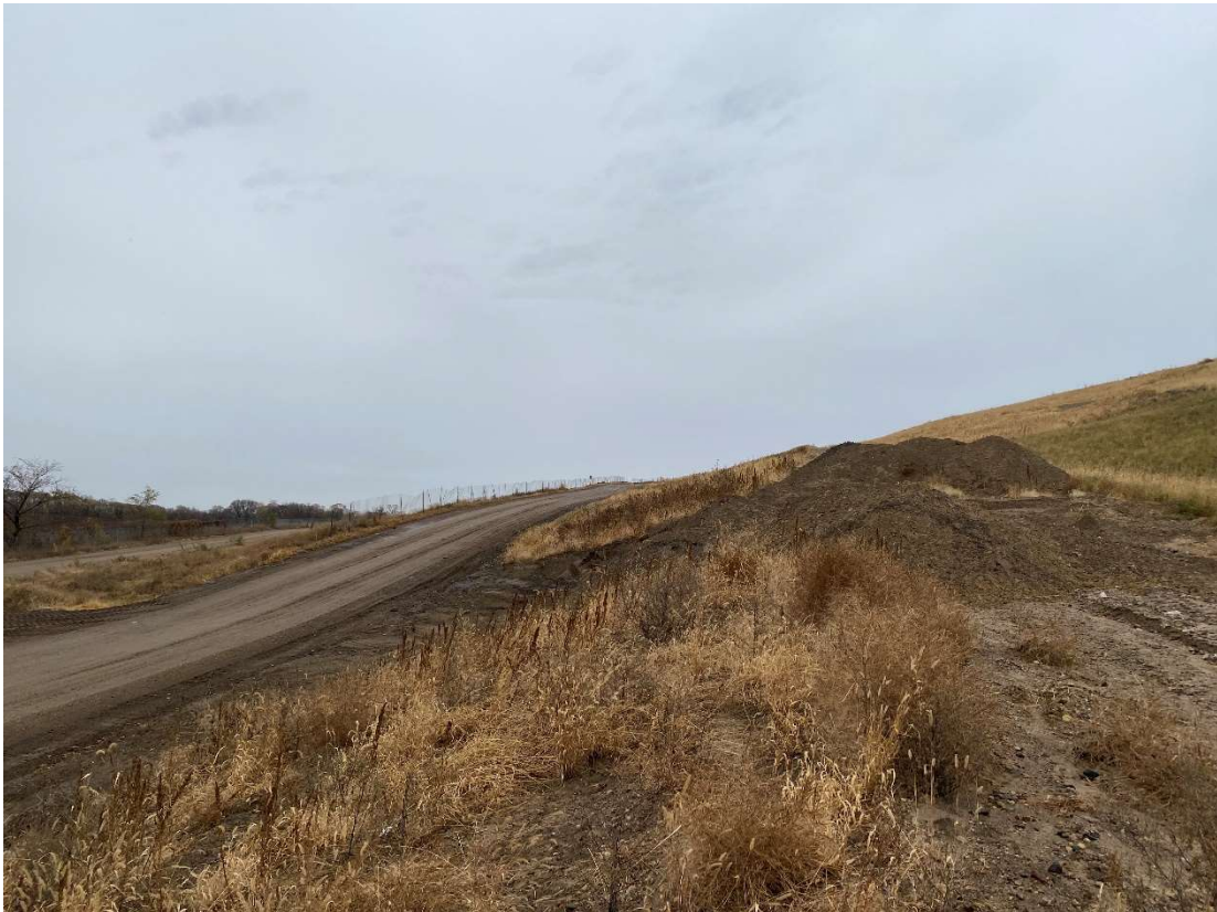
Location 3 – Looking Southwest along Cell 3 Access road/Phase 3 Liner Limit
