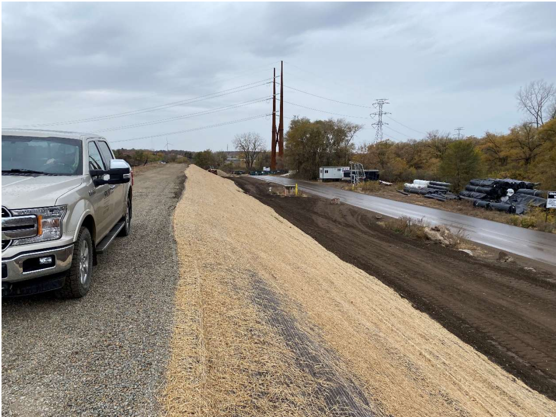
Location 12 – Cell 6A midpoint of northwestern outer berm, looking southwest
