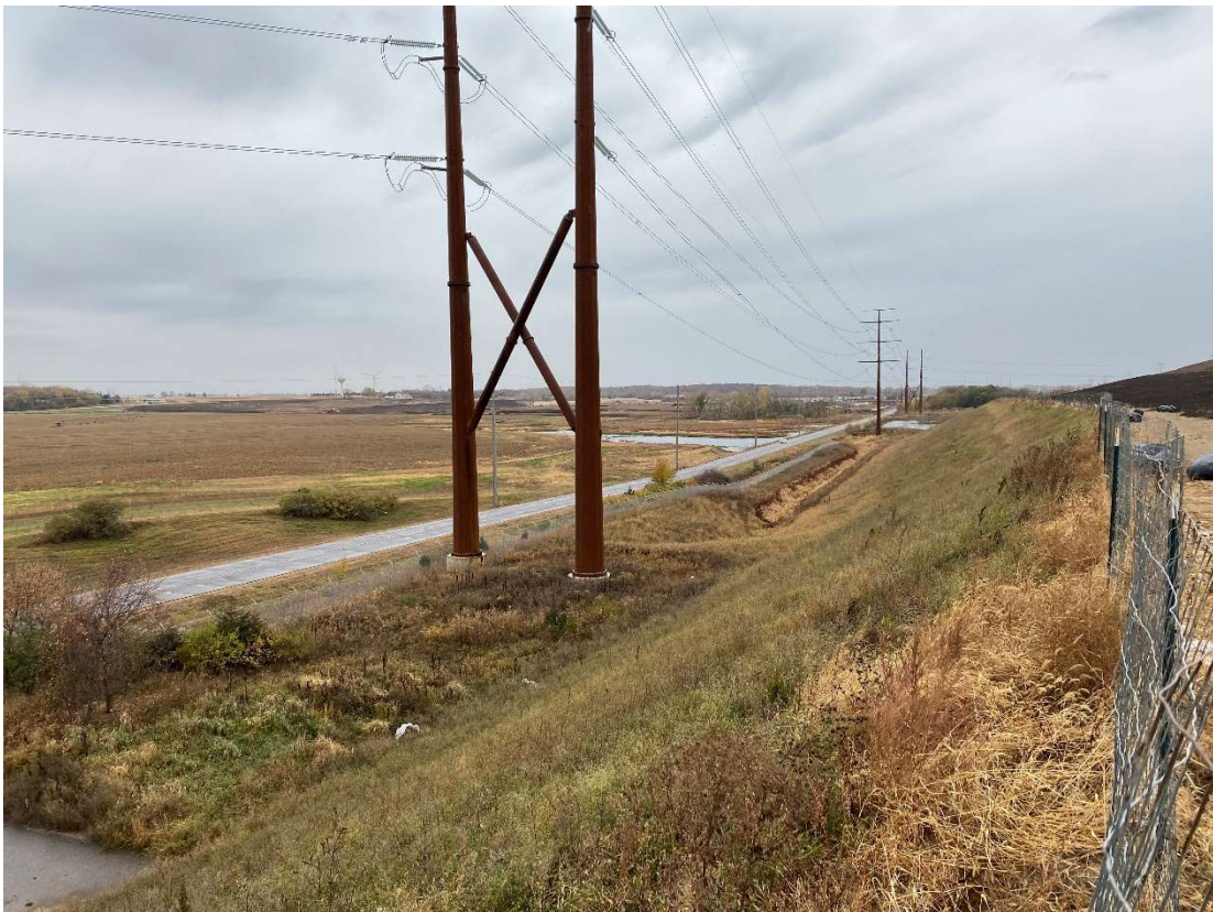
Location 6 – Cell 6D, southeast corner, outer berm, looking west
