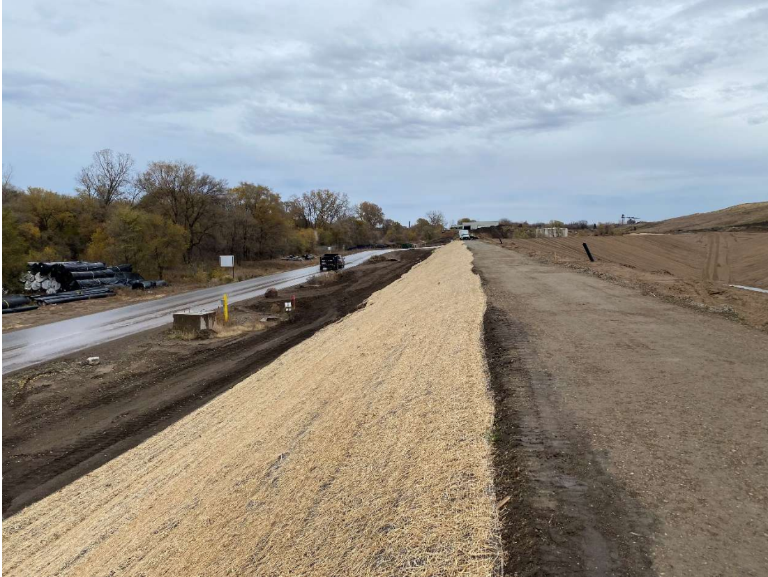
Location 11 – Cell 6A northwestern outer berm, looking northeast
