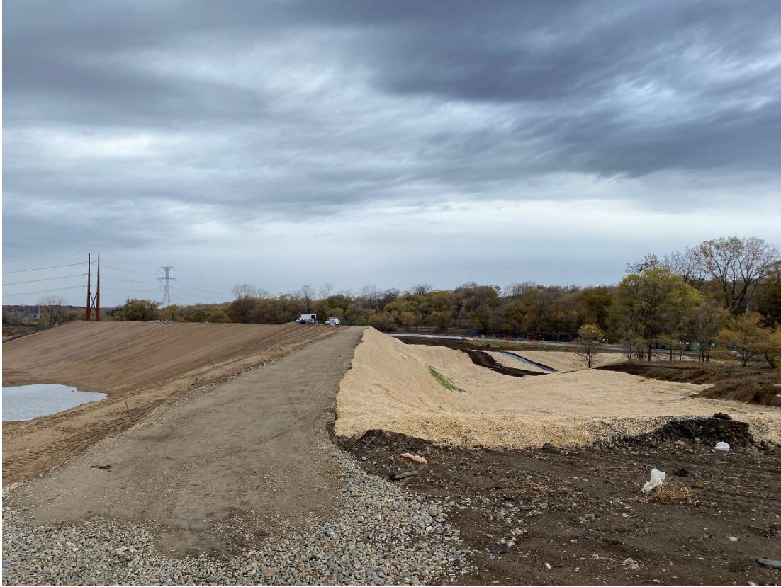
Location 14 – Cell 6A northern outer berm, looking southwest
