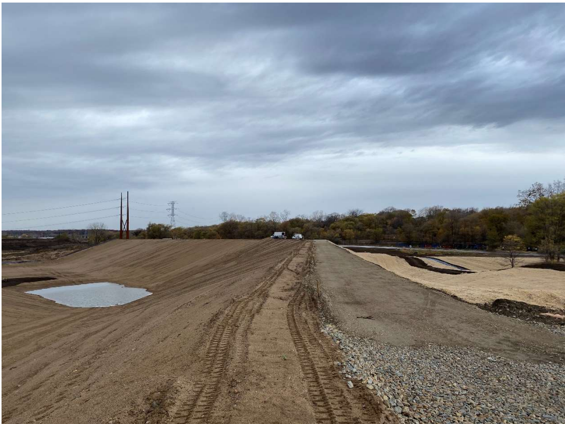
Location 14 – Cell 6A northern top of berm, looking southwest
