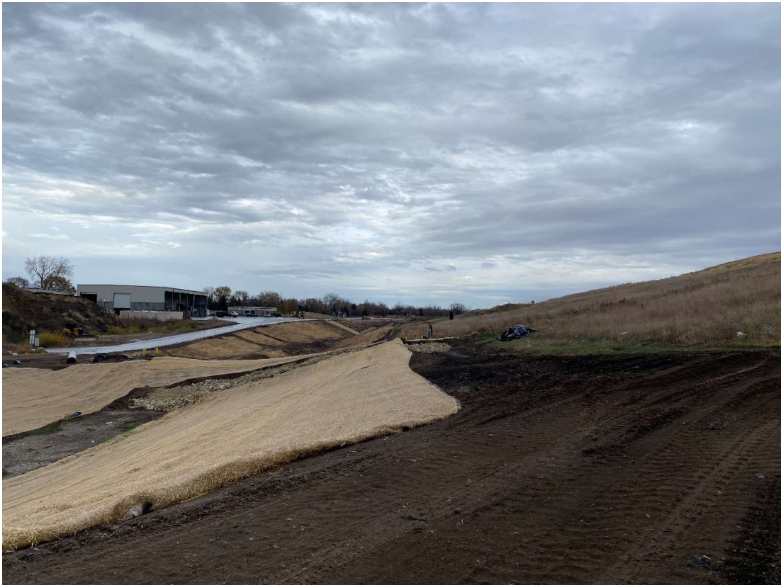
Location 14 – Cell 1 northwestern berm, looking northeast
