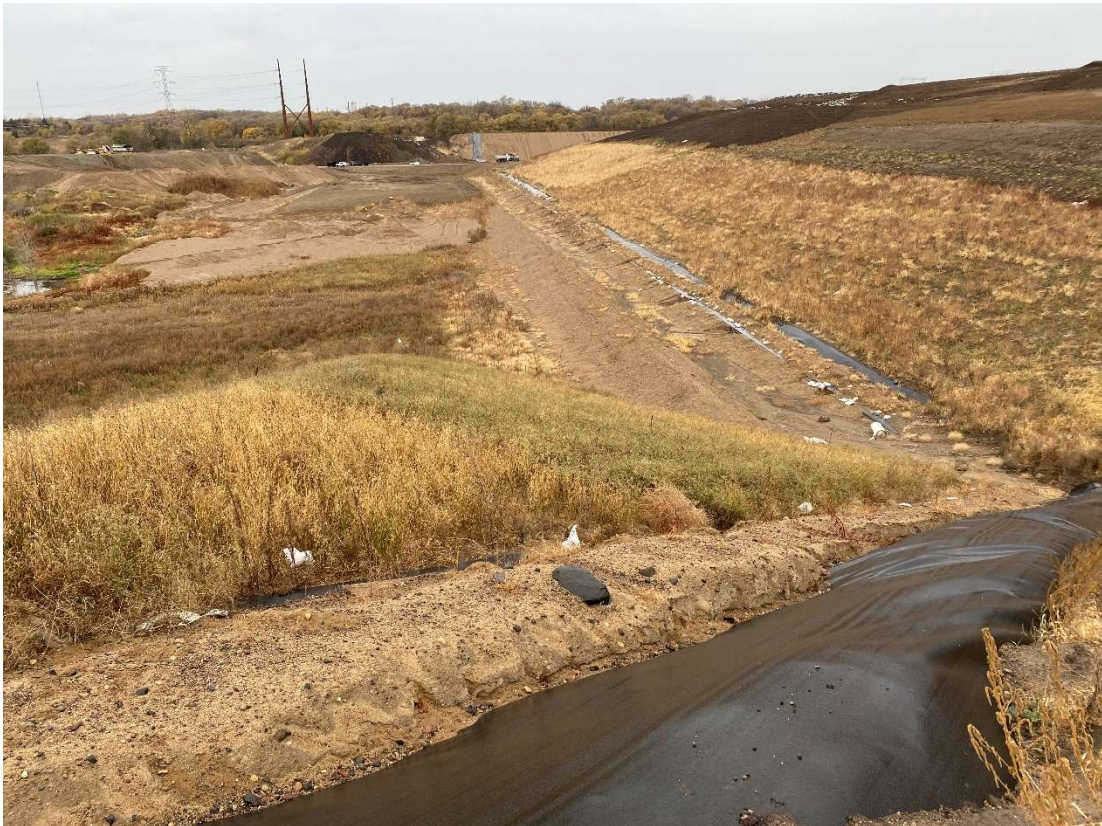
Location 8 – Cell 6D, southwest corner inner berm, looking west
