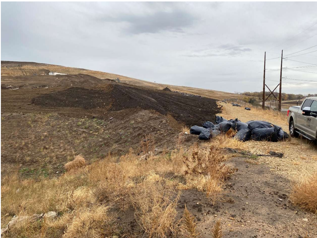
Location 8 – Cell 6D, southwest corner inner berm, looking east
