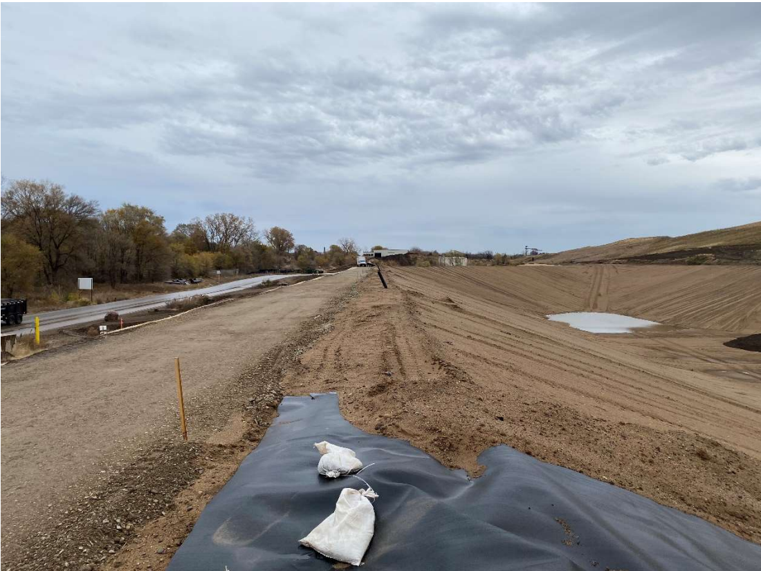
Location 11 – Cell 6A northwestern top of berm, looking northeast
