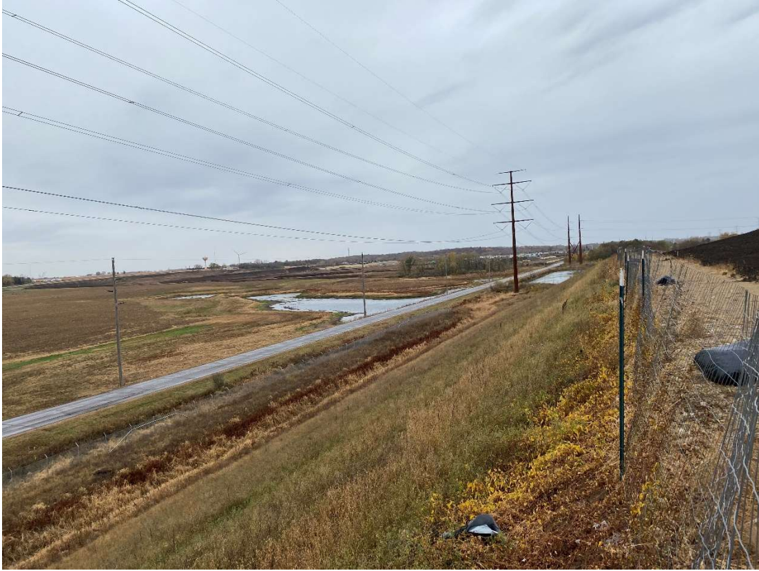
Location 7 – Cell 6D, midpoint of outer berm, looking west
