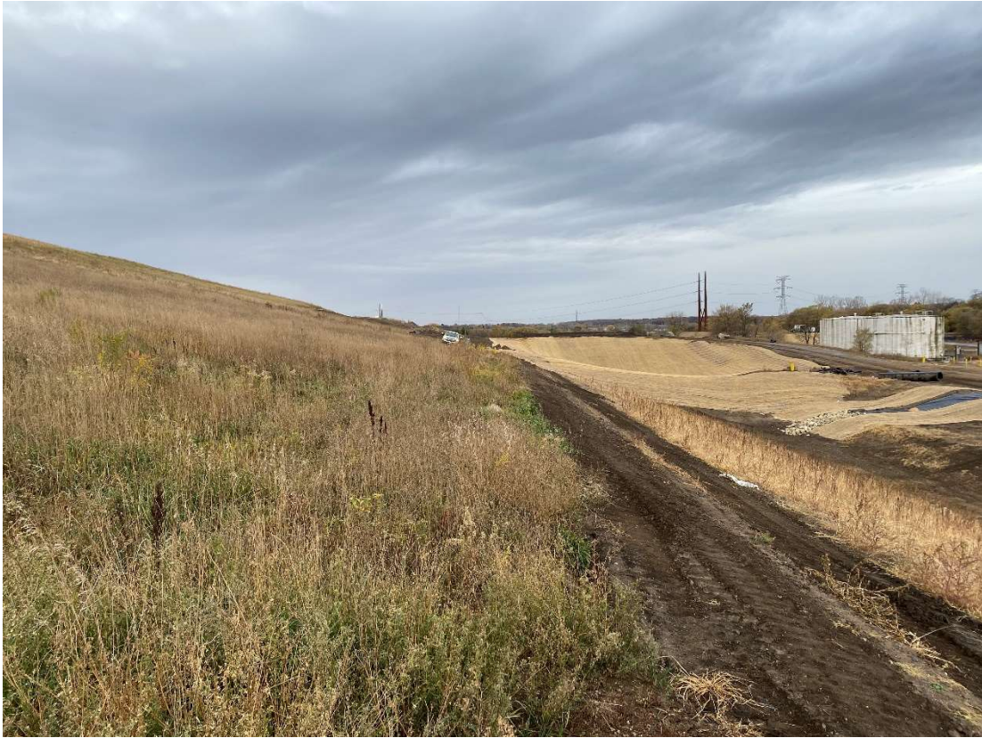
Location 15 – Cell 1 Toe of Waste Slope, looking southwest
