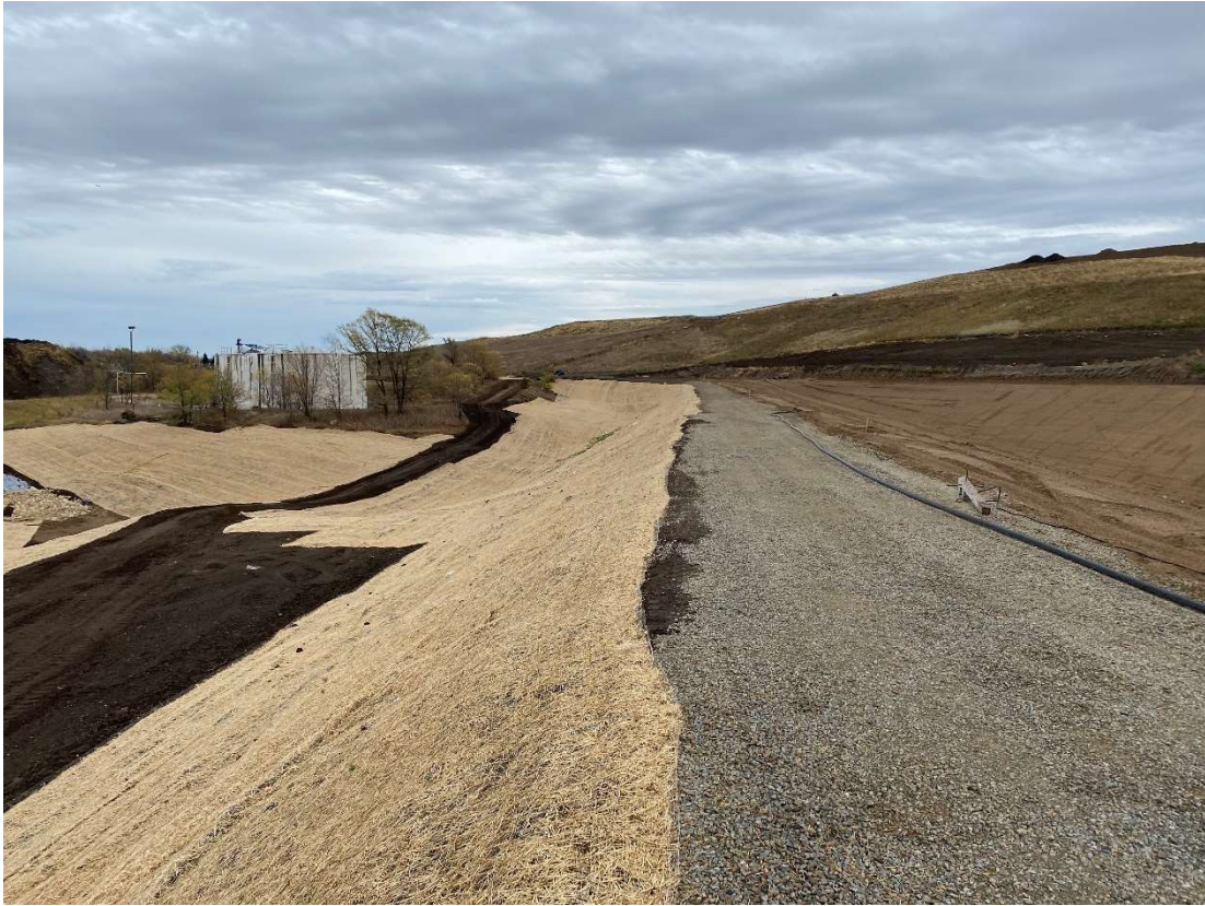
Location 13 – Cell 6A northern outer berm, looking northeast
