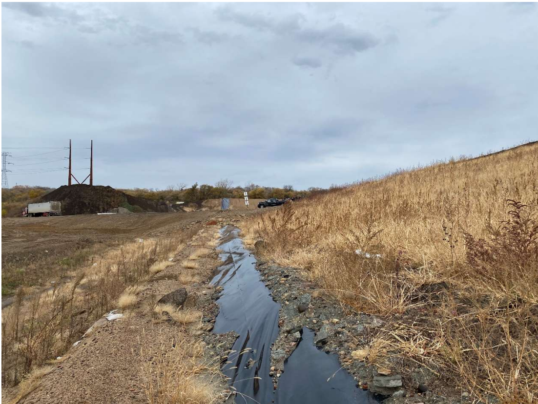
Location 10 – Cell 6A southwestern limits, looking northwest
