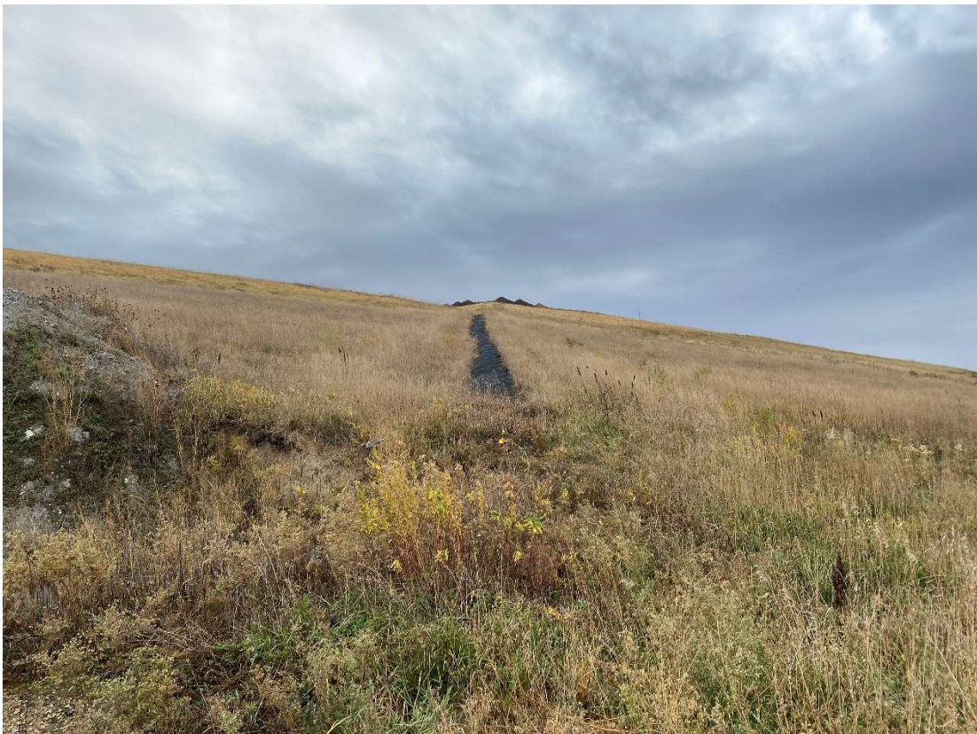
Location 15 – Cell 1 edge of cap, looking south
