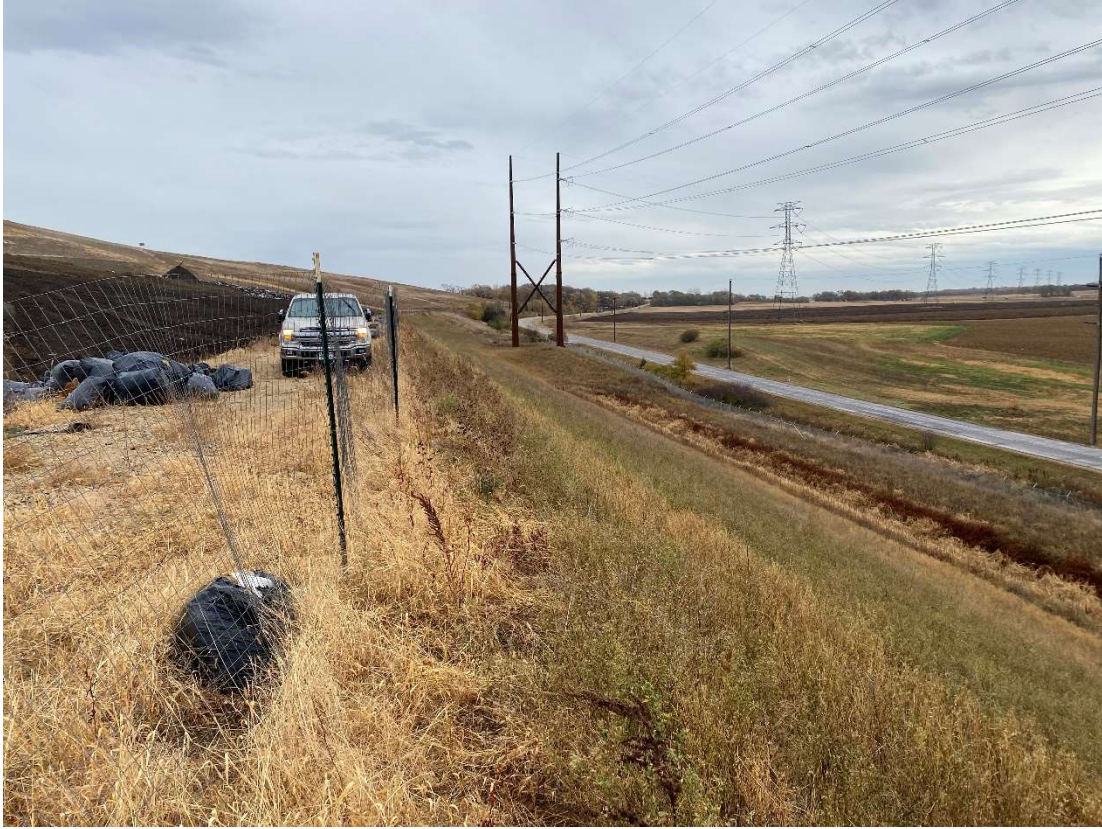
Location 8 – Cell 6D, southwest corner outer berm, looking east
