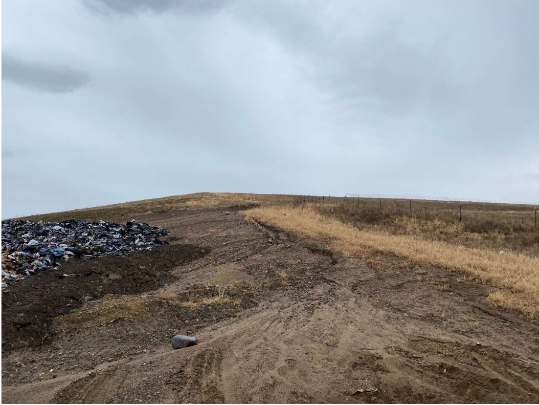
Location 6 – Cell 6D, southeast corner, looking northwest
