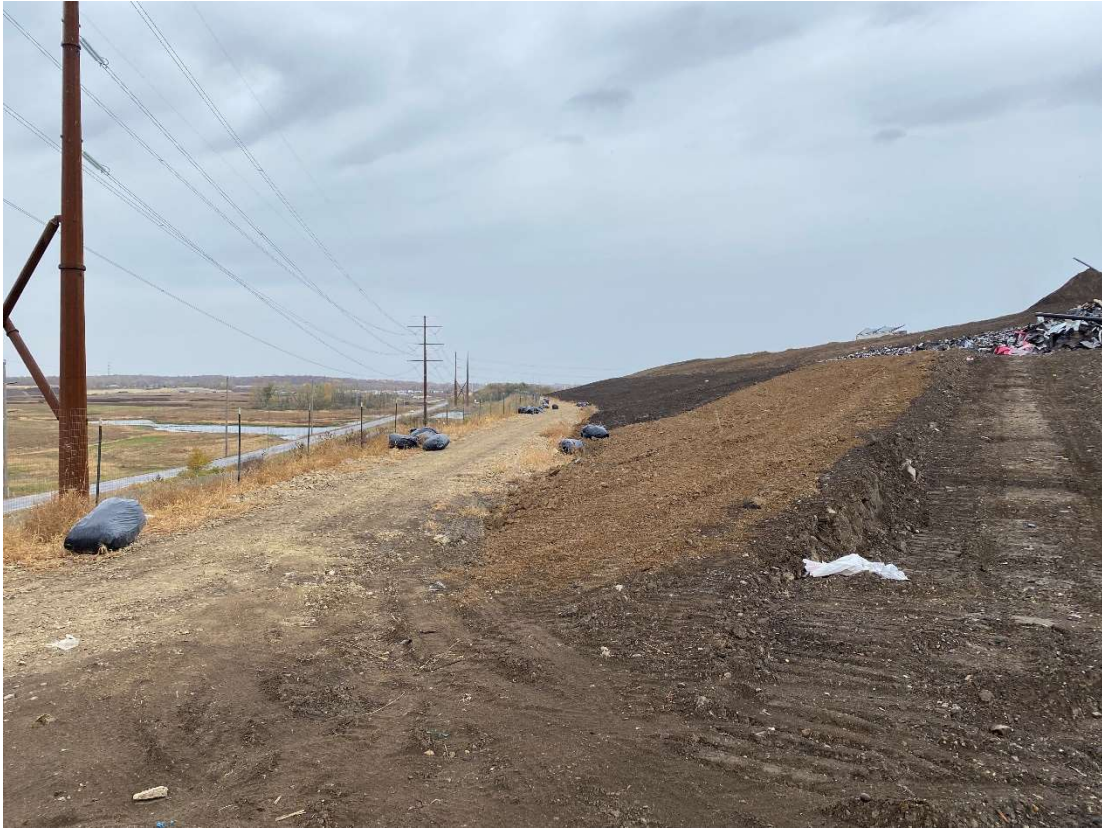
Location 6 – Cell 6D southeast corner, inner berm, looking west
